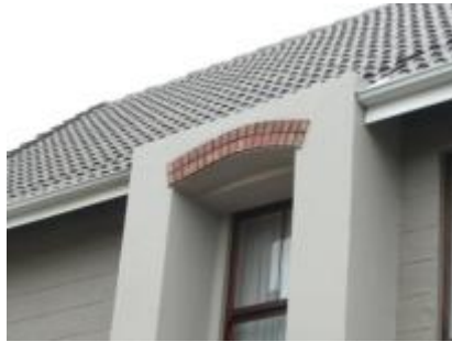
Red Face Brick Plinths
