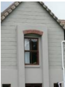
Typical External Wall finish to Second Level
