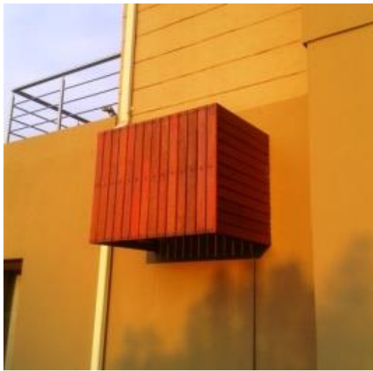
Air Conditioning motor unit hidden behind Metal frame and Timber Slat air conditioner compressor
